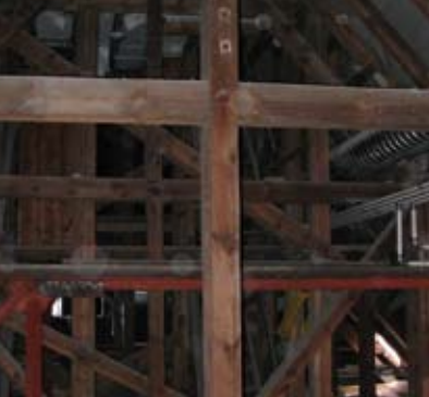
Roof construction, Germany
